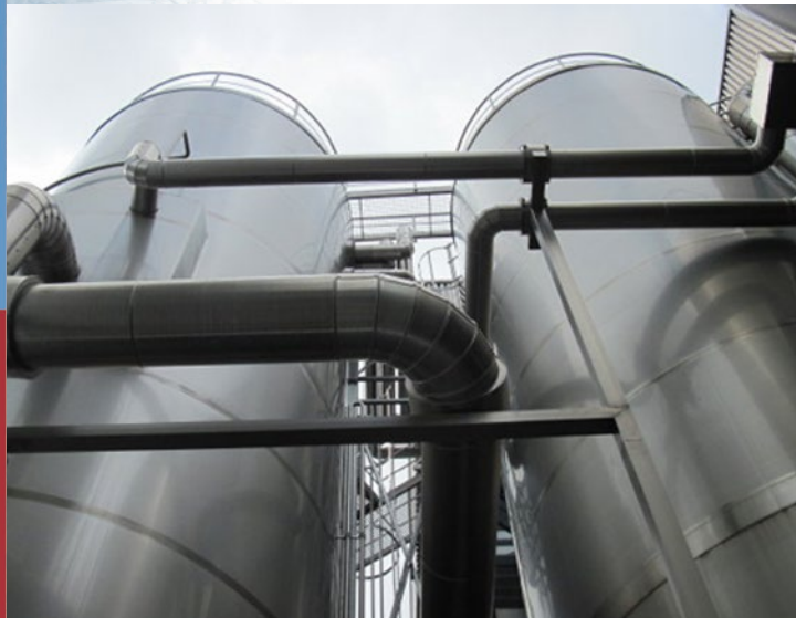
PIC LEFT ice silos with 5000 kWh storage capacity each PIC RIGHT ice maker for 6 to/h. At 10 h buildup time 5600 kWh
